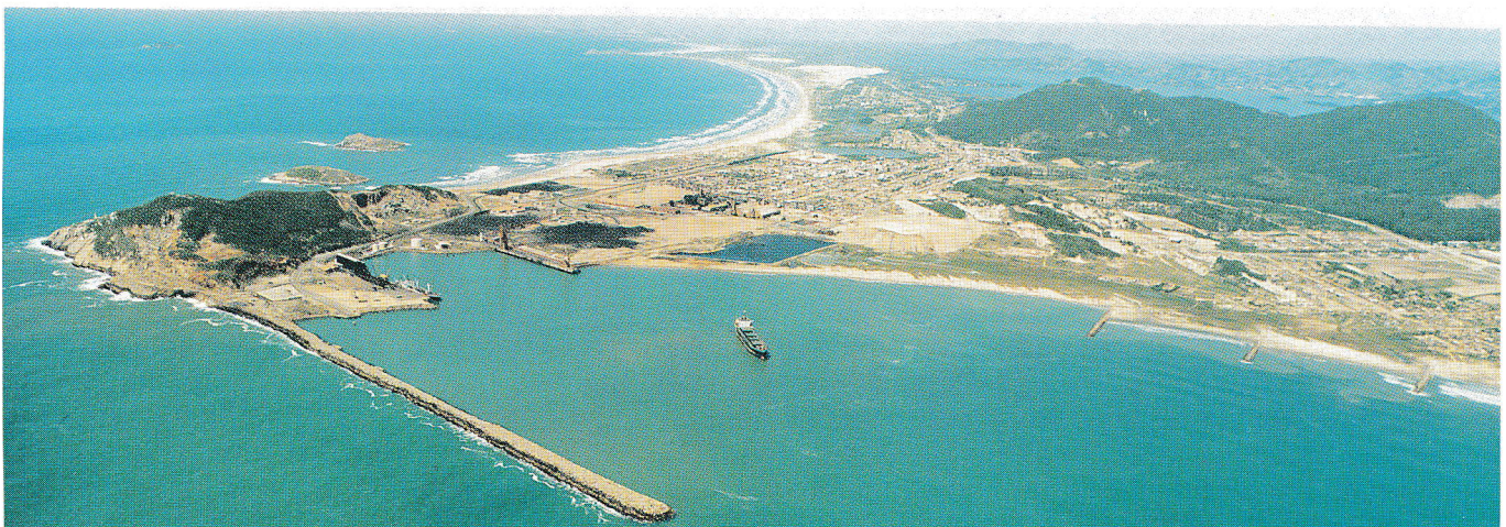
- Imbituba, a private port in Brazil
